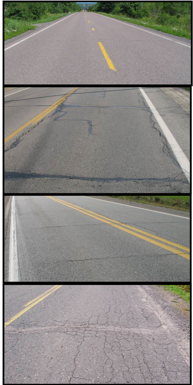
Figure 1: PASER Road Ratings. Top image, above – PASER 8 road that is considered “good” by the TAMC and exhibits only minor defects. Second image, above – PASER 5 road that is considered “fair” by the TAMC and exhibits structural soundness, but could benefit from CPM. Third image, above – PASER 6 road that is considered “fair” by the TAMC. Bottom image, above – PASER 2 road that is considered “poor” by the TAMC exhibiting significant structural distress.
